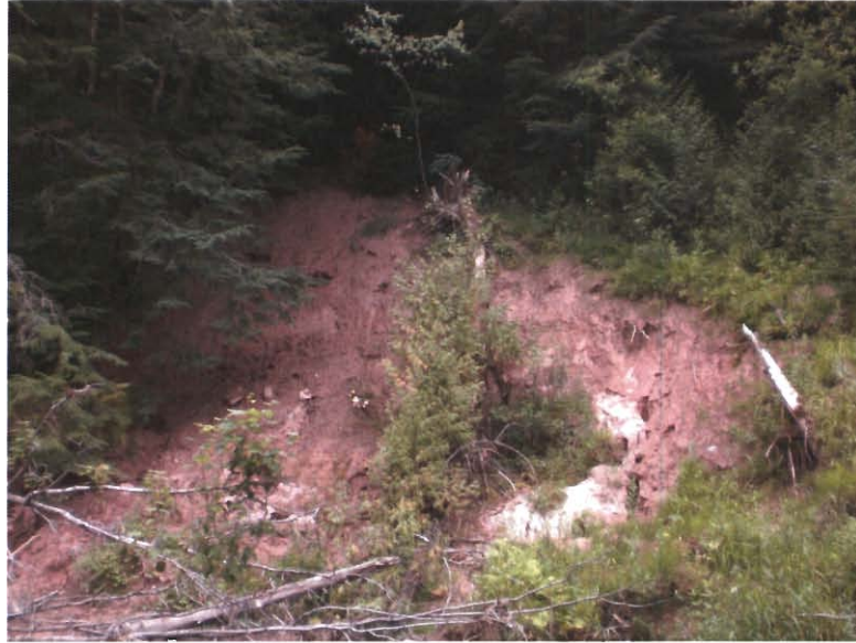
Figure 39: Erosion Site Four
