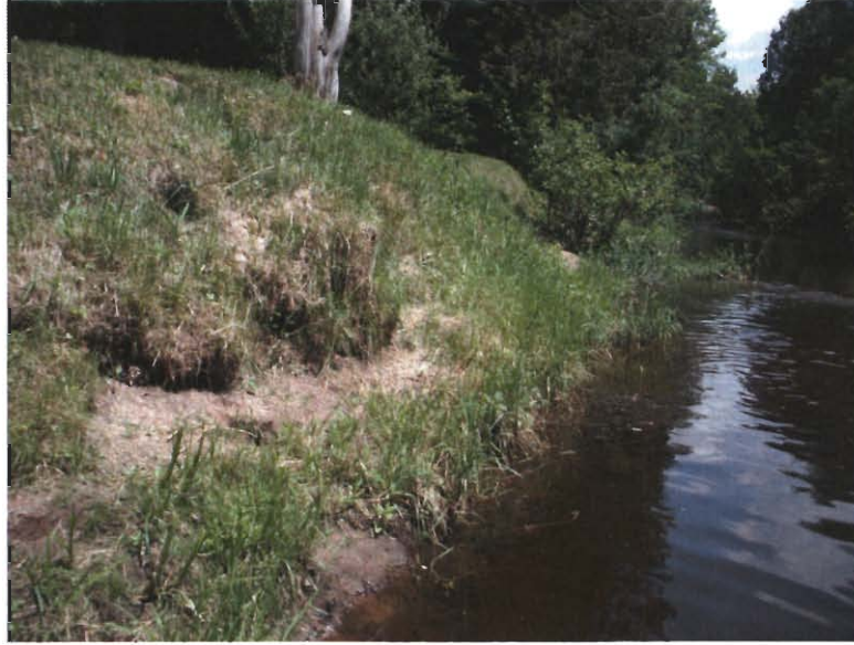
Figure 48: Erosion Site Thirteen
