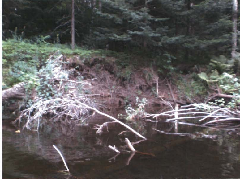
Figure 42: Erosion Site Seven
