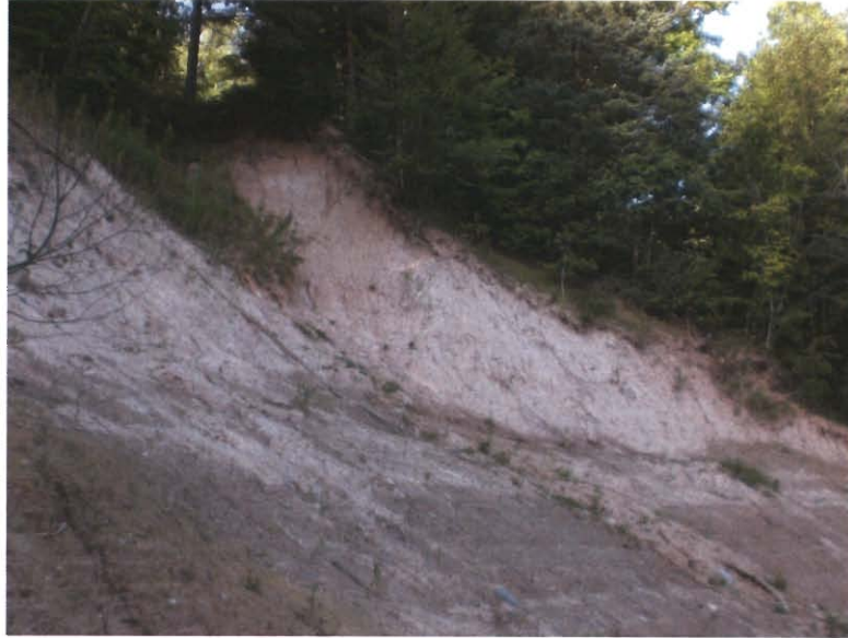
Figure 36: Erosion Site One
