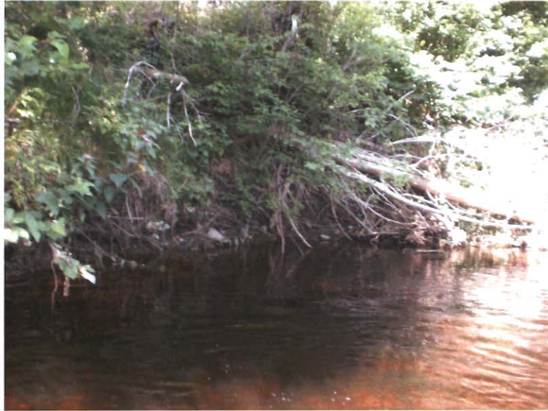
Figure 45: Erosion Site Ten
